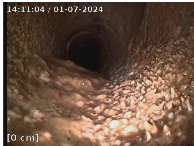
Thick layer of deposits
