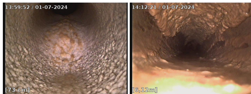
Figure 4.5 Thick layer of deposits at inspection point 14 (left) and 15 (right)
