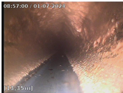
Figure 4.2 'Highway pattern' in the pipe segment inspected from point 2 towards point 1
