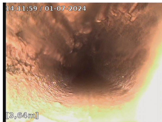
Thick layer of deposits
